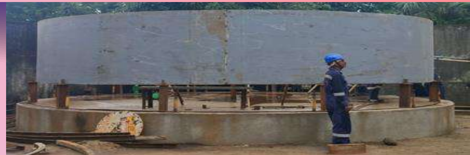
75 KL TANK FABRICATION
