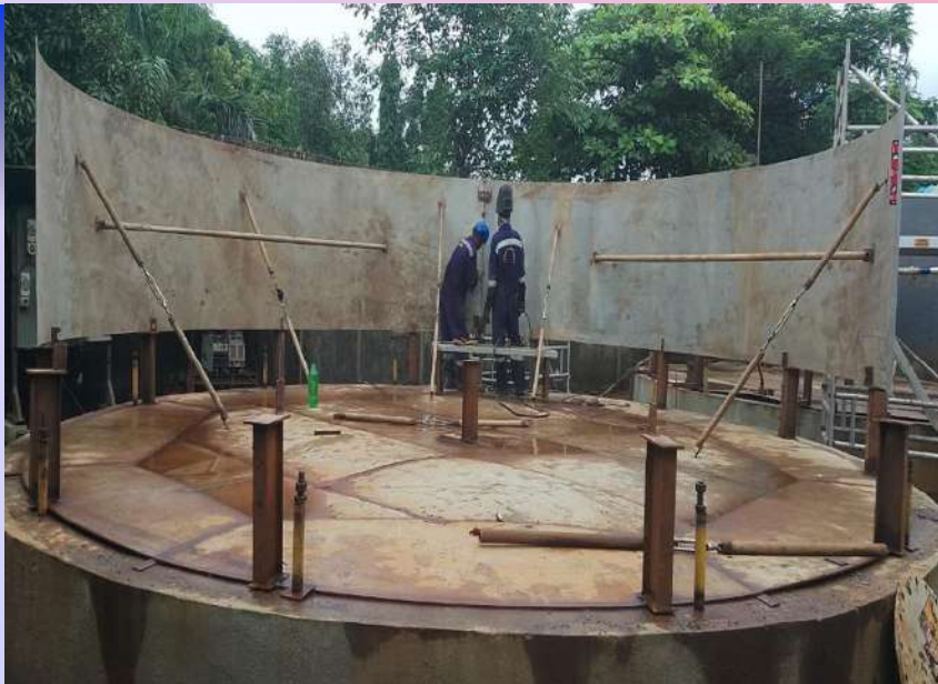
450 KL TANK SHELL FABRICATION
