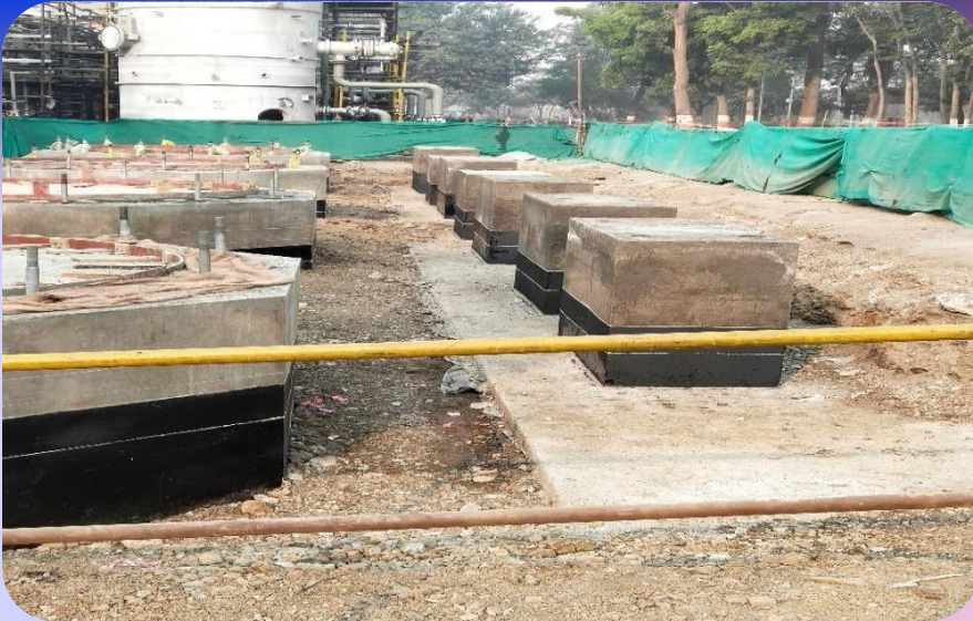
TANK FOUNDATION & PUMP FOUNDATION
