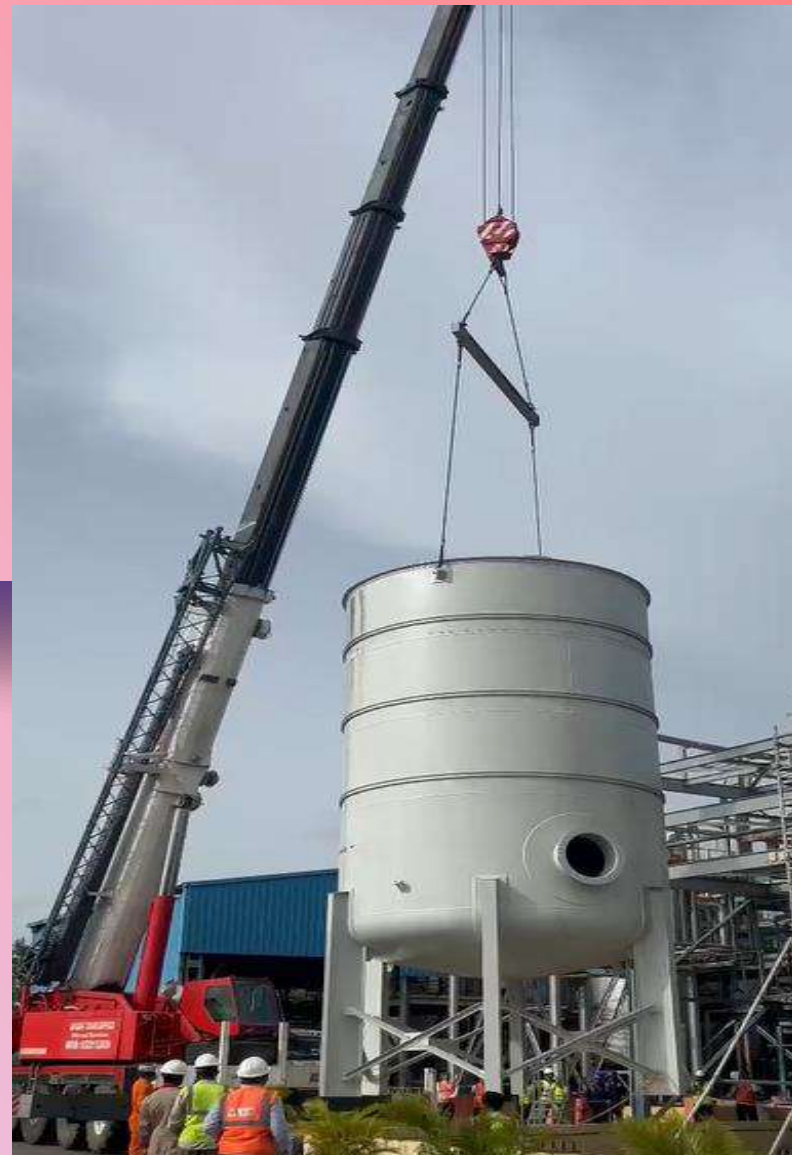
100 KL TANK ERECTION
