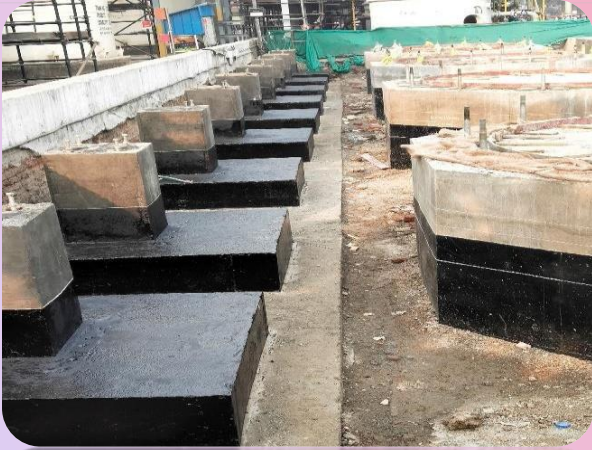
PIPE SUPPORT FOUNDATION
