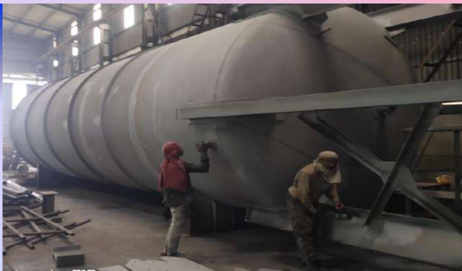
100 KL SHELL FABRICATION
