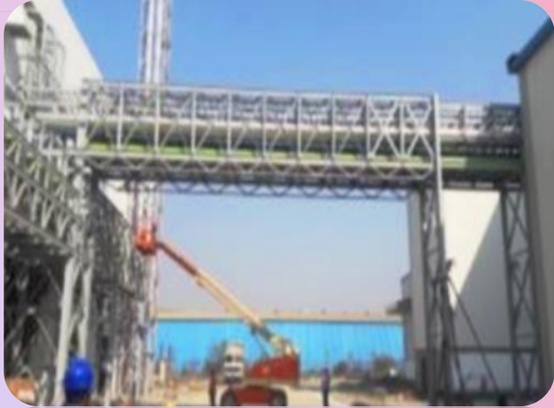
PIPE RACK STRUCTURE
