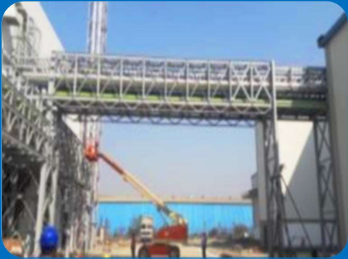
PIPE RACK STRUCTURE
