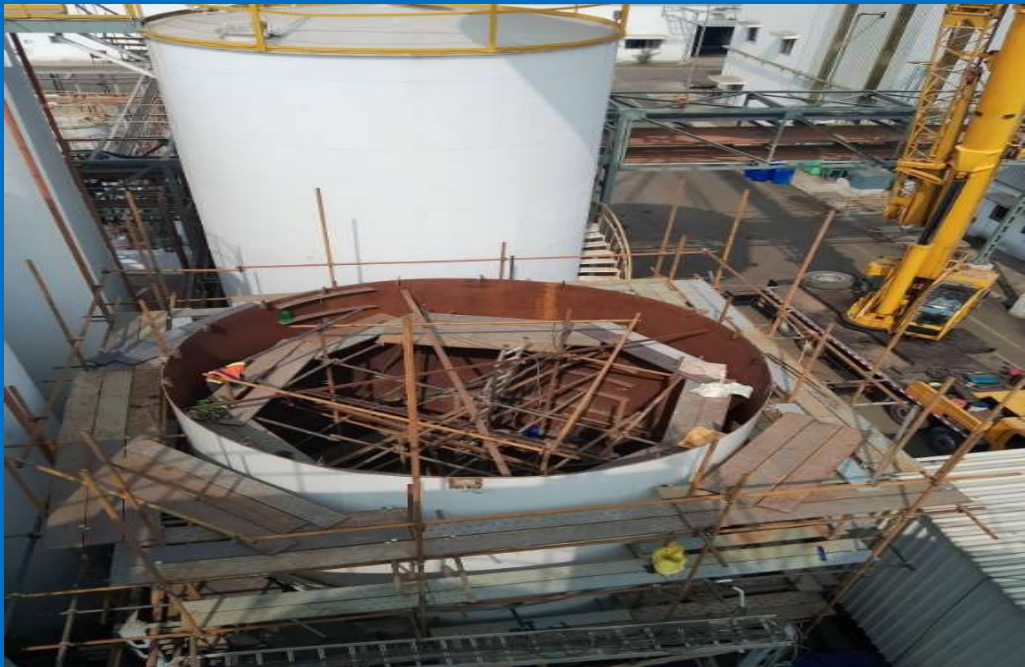
300 KL TANK FABRICATION & ERECTION
