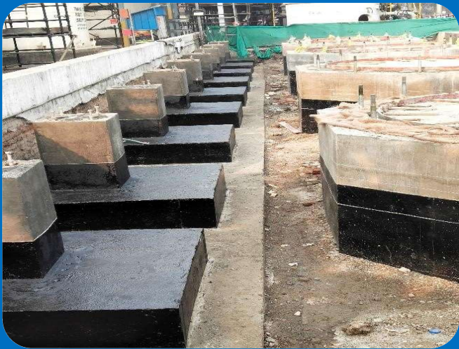
PIPE SUPPORT FOUNDATION
