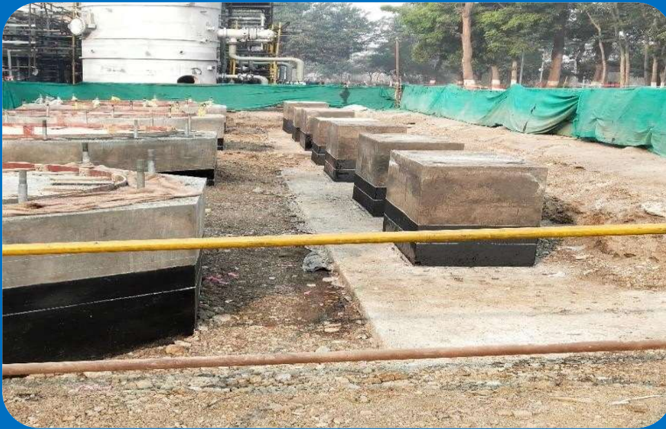
TANK FOUNDATION & PUMP FOUNDATION
