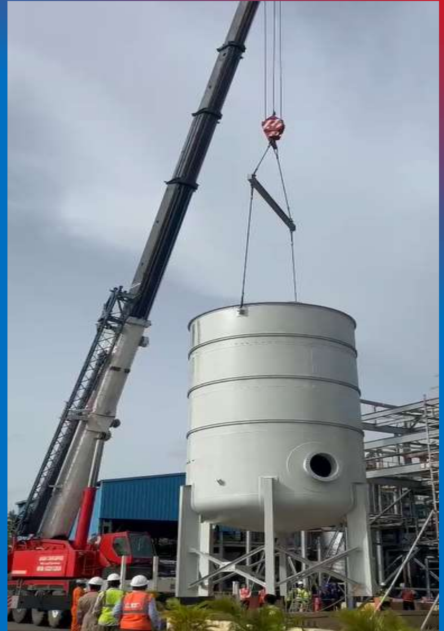
100 KL TANK ERECTION
