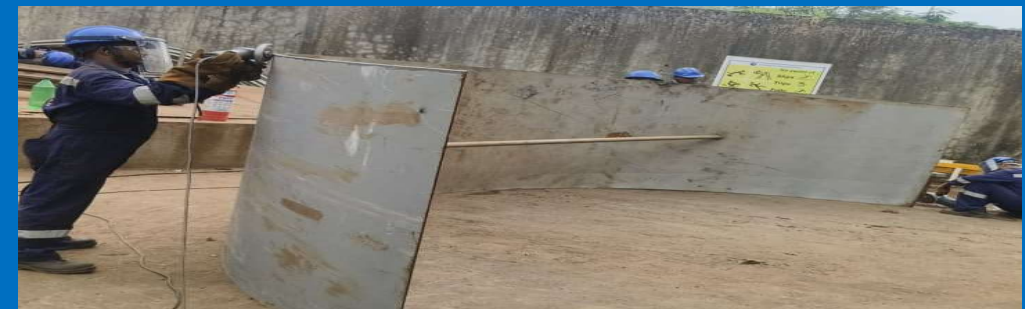
450 KL TANK SHELL FABRICATION
