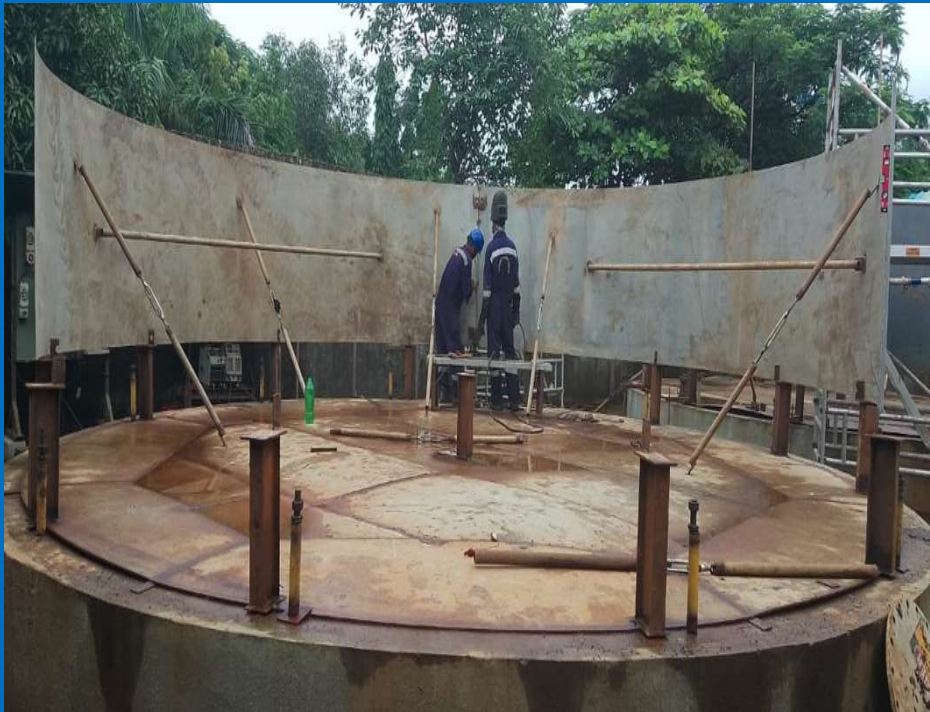
450 KL TANK SHELL FABRICATION
